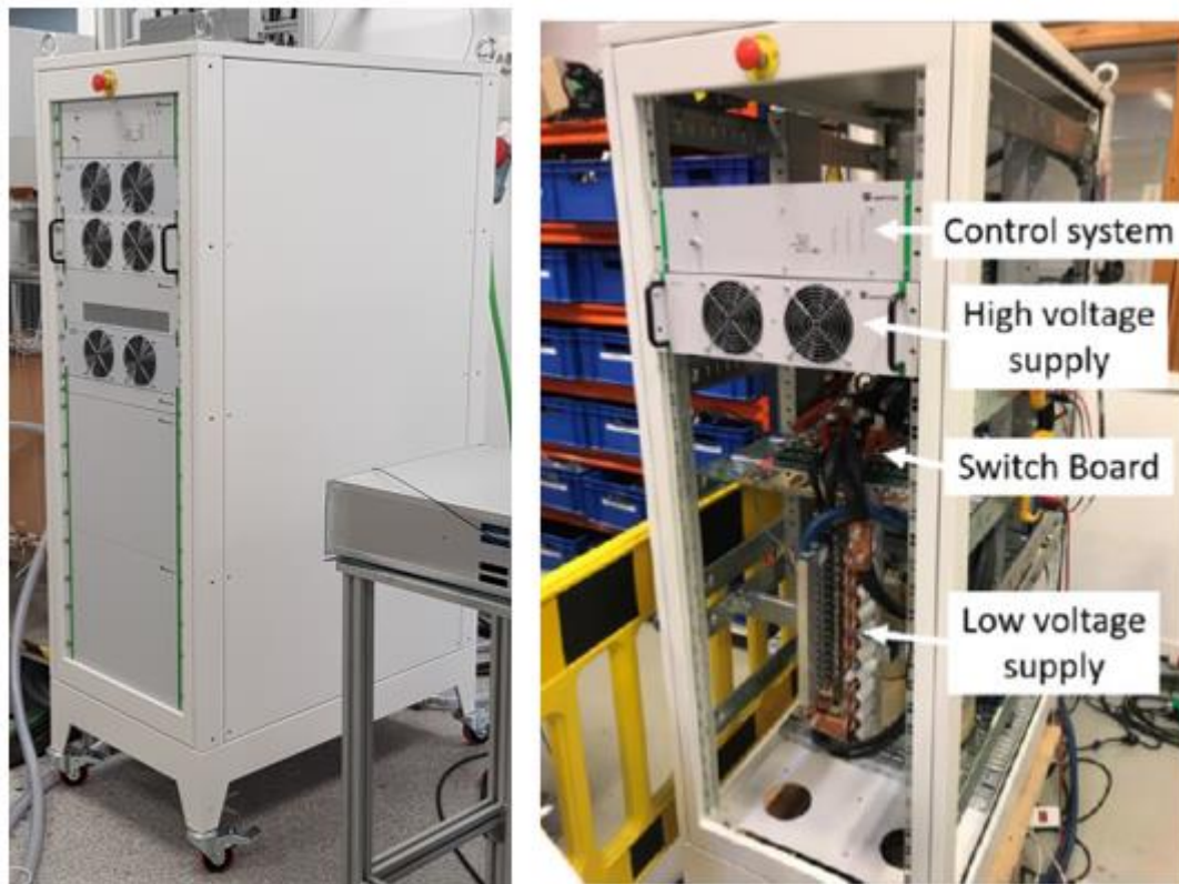
Figure 8: (Right) Picture of the Danfysik PPSU. (Left) Picture of the main components.
